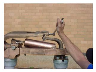
Figure 4: Switch Adjustment in Open Position
