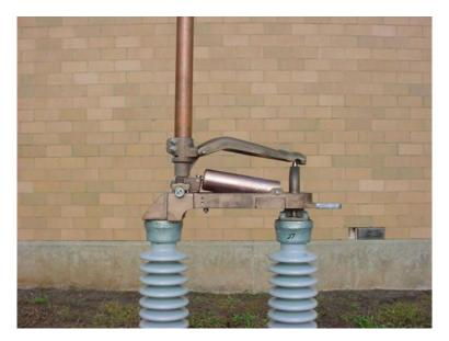
**Figure 3: Stack Insulators**
